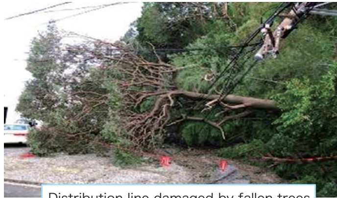
Distribution line damaged by fallen trees
